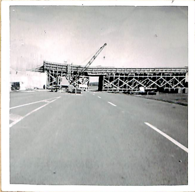
Building 401 overpass Bridge at Shannonville Road
