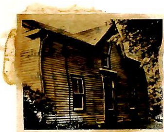
House before restoration
