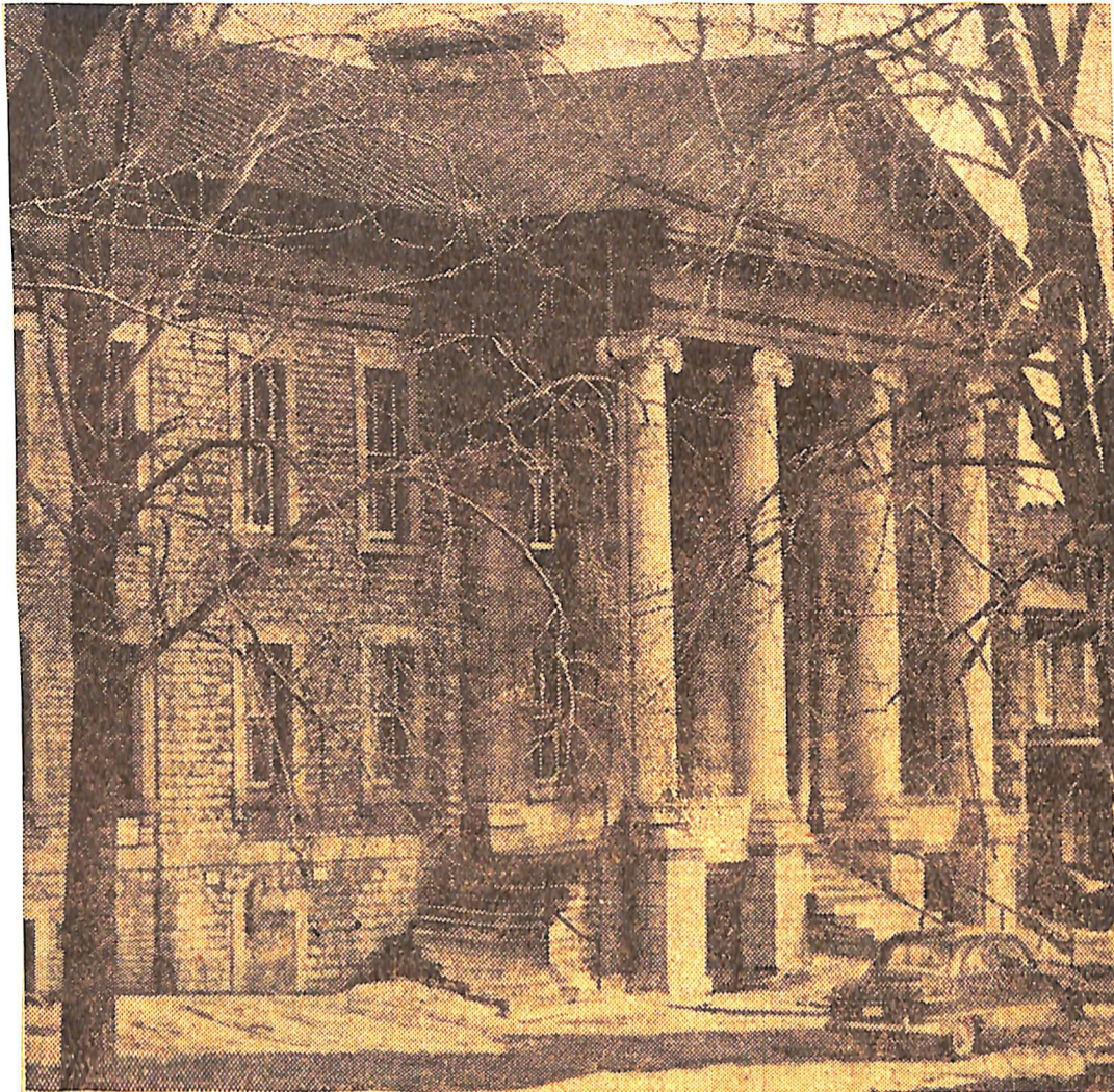
HASTINGS COURT HOUSE, 1839 —Above pillars of 120-year-old Hastings county court house, have already disappeared and court house itself will eventually go under the wreckers' hammer
