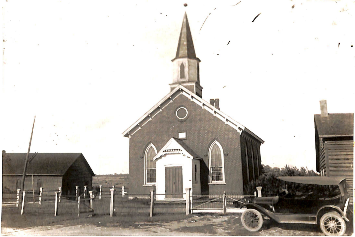
Bethel church - built 1863. Building at left is Forester's Hall Building at right is Post Office. The 1916 Chevrolet in the foreground belonged to Ben. Sayers, father of Earl Sayers.
