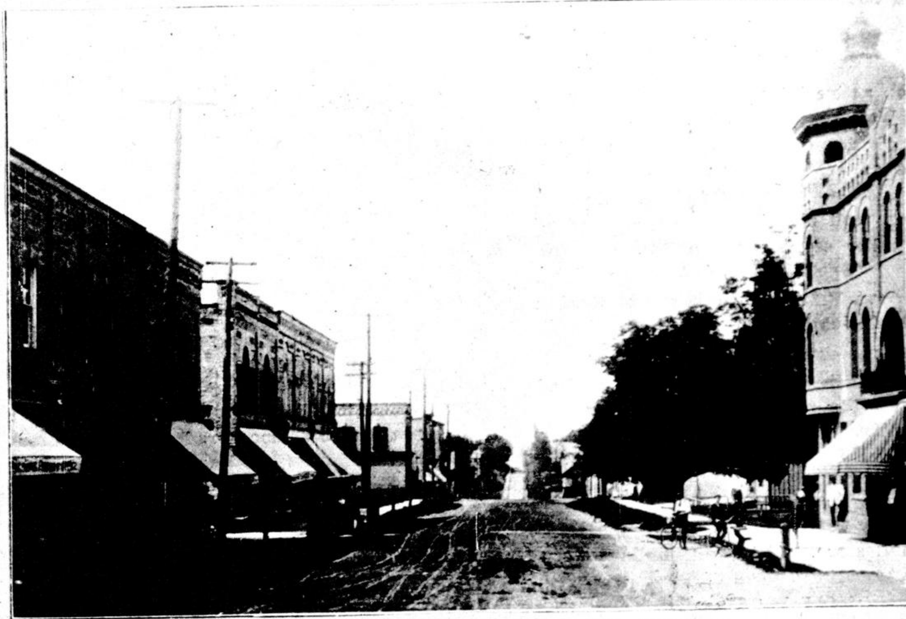
CLINTON STREET LOOKING NORTH
