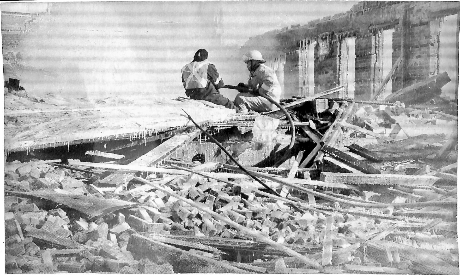
Ruins of Russell's Commercial Hotel after fire January 10, 1991.
