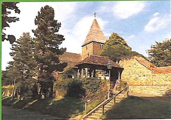
St. Peter's Church. Limpsfield.
