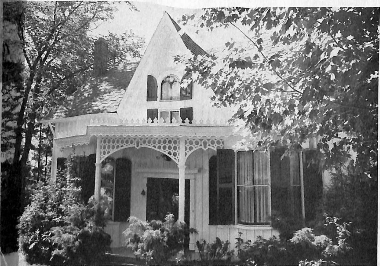
Pictured above is the new verandah on the Erland Lee Home, replica of the original. The front doors also were restored to their original style.
