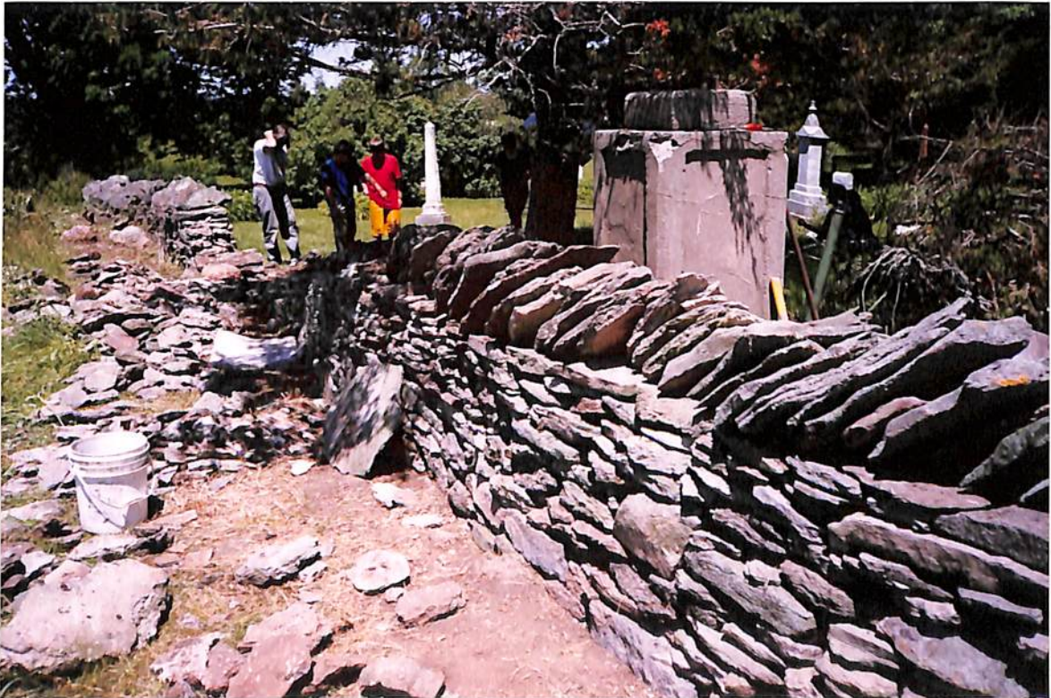
The first section to the concrete pillar completed
