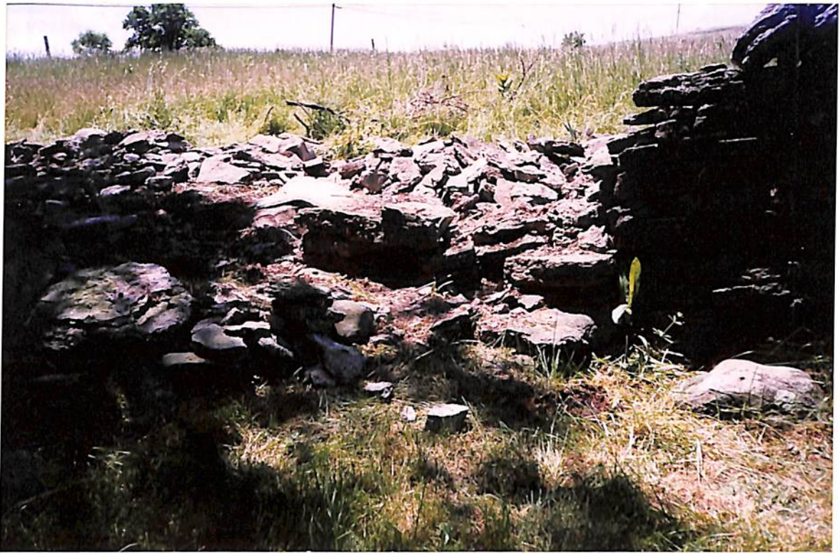
Dismantling the fence
