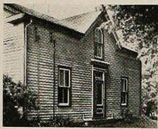
House before restoration.
