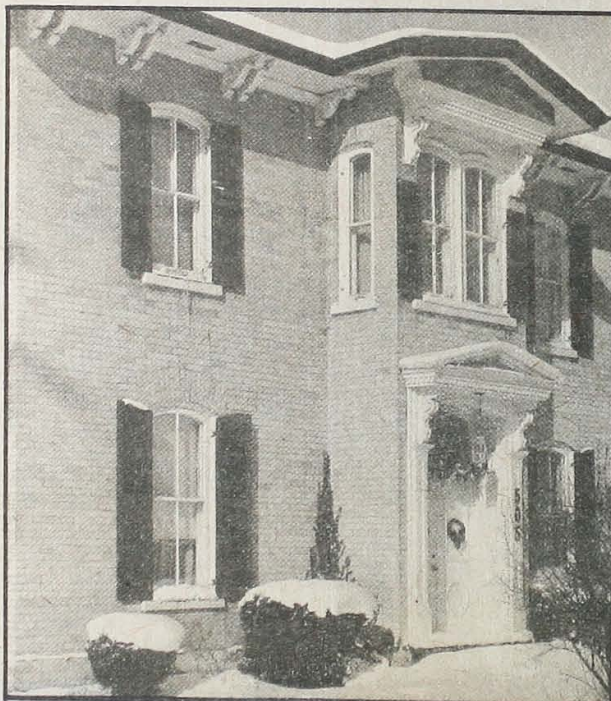
THE RAREST EXAMPLE of the Italianate style in the province, including the projecting frontace piece, is found in the Alton house which is located on Colborne Street. (Stull photo)
