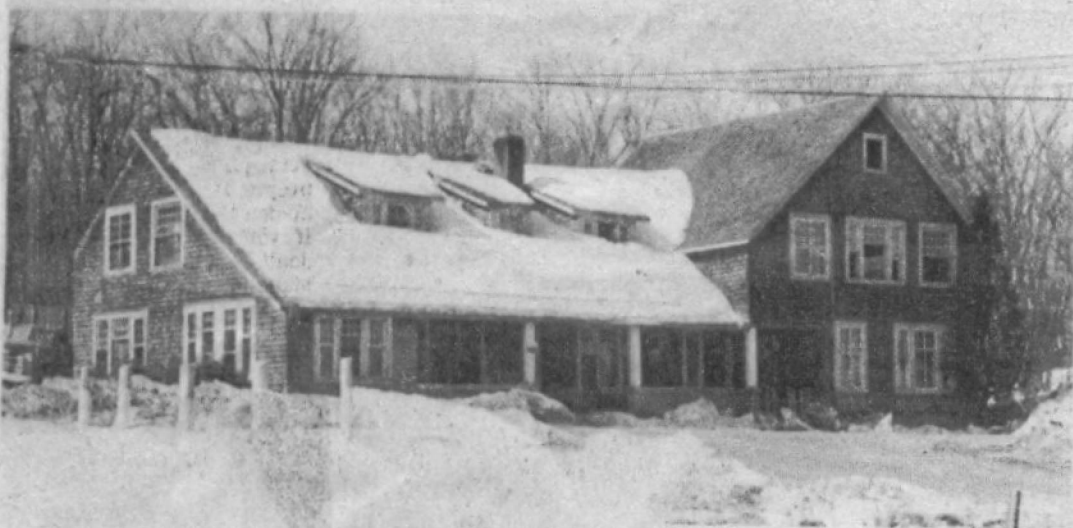
WINTER'S JUST FADING as this photo was taken of the Braeside Inn as demolition was
