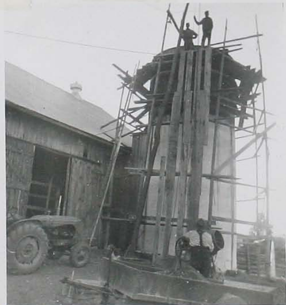
Silo Building - Oval Crispin
