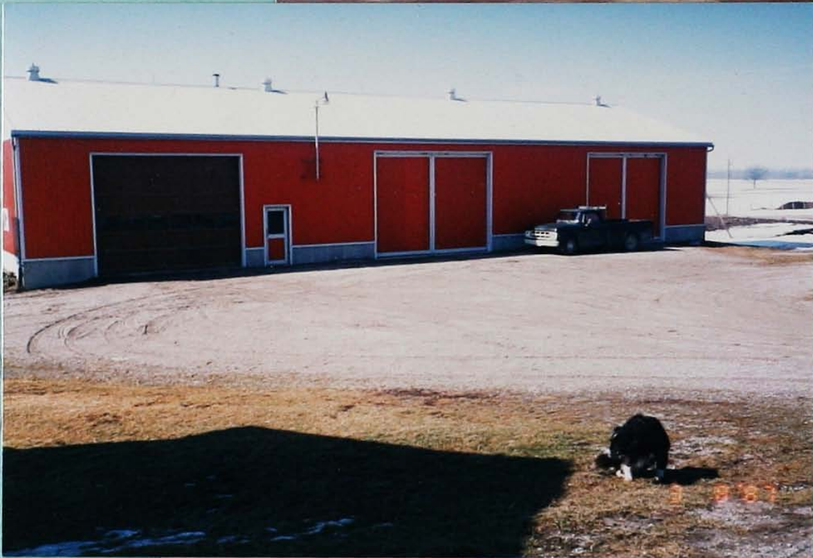
Steel Shed built by Raph Poehman in 1972.
