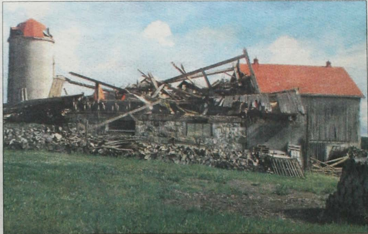
Bryan and Margaret Crispin's barn, located on the outskirts of Brockton near Hanover, was destroyed by a tornado that touched down in the area last Tuesday. Environment Canada reported winds reached speeds of between 160 and 180 kilometres per hour.
