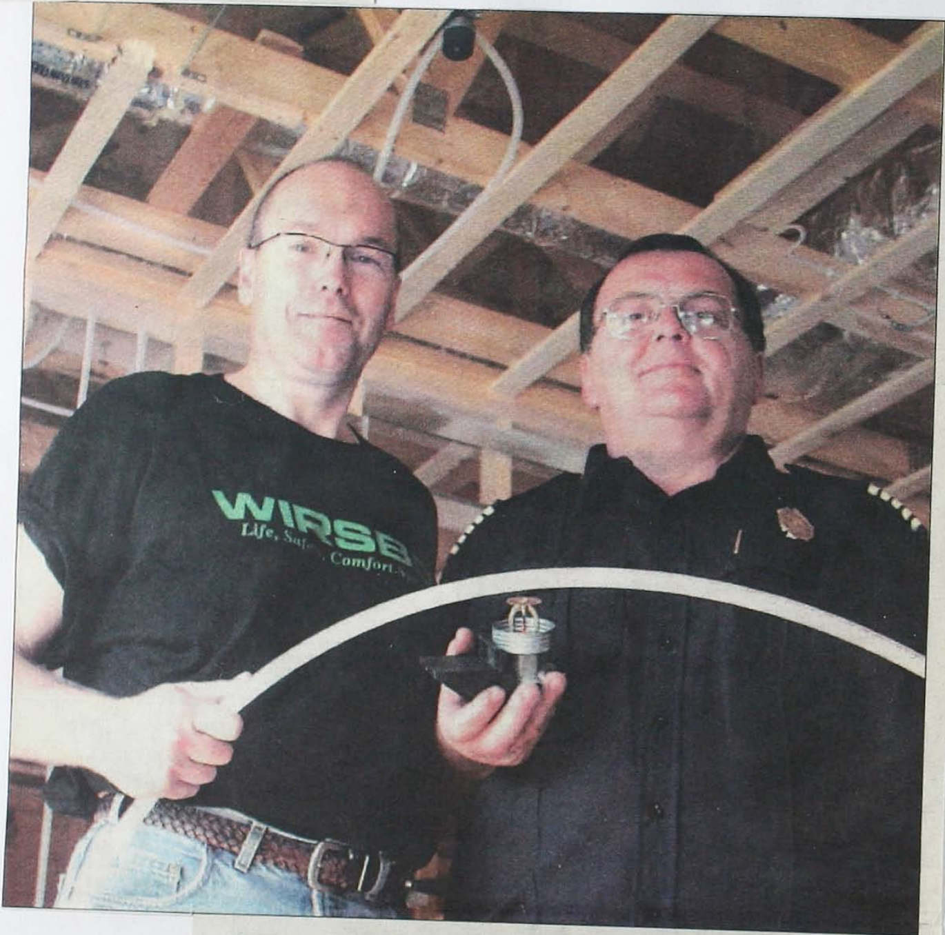
Walkerton Fire Chief Ken Freiburger, right, holds up one of many sprinkler heads being installed in his new home, while Kevin Price of Uponor Canada Inc., shows off the flexible tubing his company uses to install residential sprinkler systems. The systems are fairly new to the residential market.
