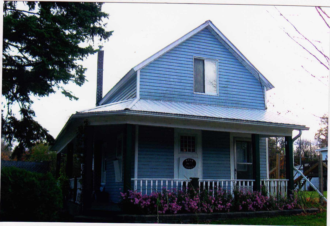
One of the older homes with a lovely veranda addition
