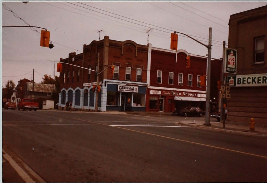
Oct. 1979 Installation of Traffic lights
