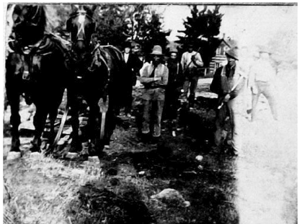
Doing repair work on the road through Glasgow
