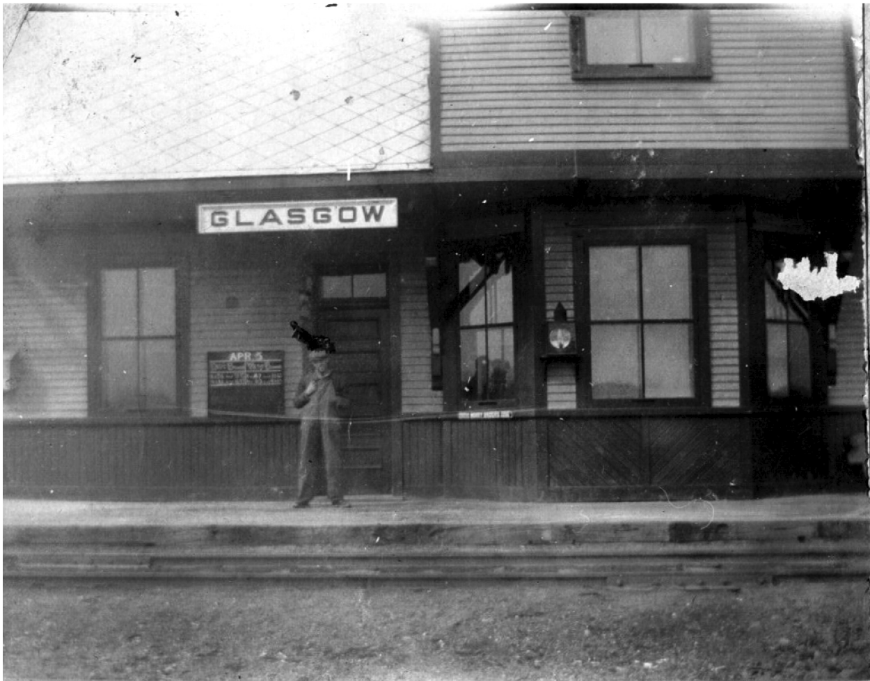
Glasgow Station which was destroyed by fire. Mr. H. Johnston, agent is standing in front
