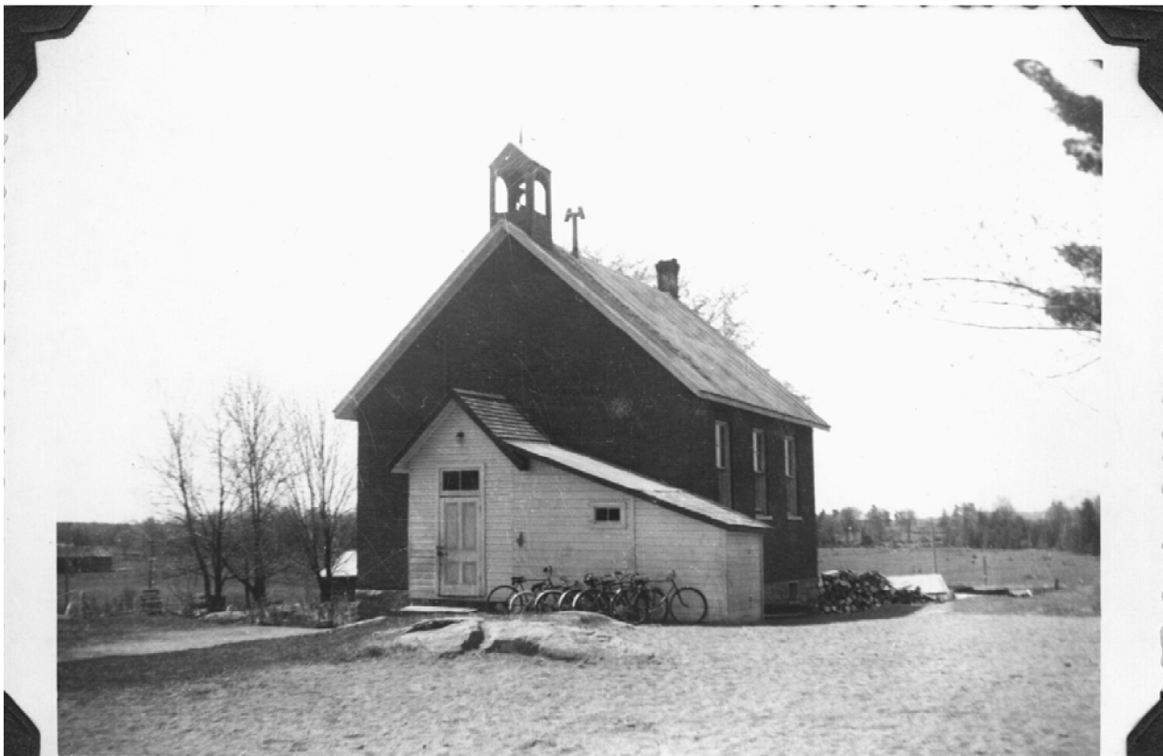
School built 1905. Photo 1953
