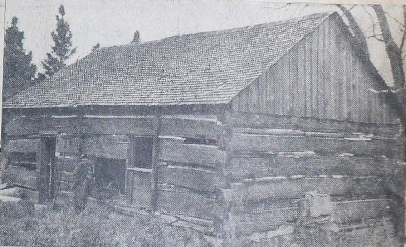
POSSIBLE AMABEL MUSEUM — Stan Smith, a farmer in Amabel township and a former trustee and secretary-treasurer of S.S. No. 10 in the township, looks over the second school built in Amabel. His father helped build it in 1873 and it has been abandoned
