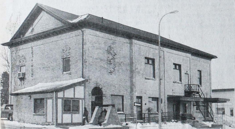
By the 1990's the town hall, now a historical building, has lost many of its original features. The Local Architectural Conservation Advisory Committee would like to see the exterior of the town hall restored.
