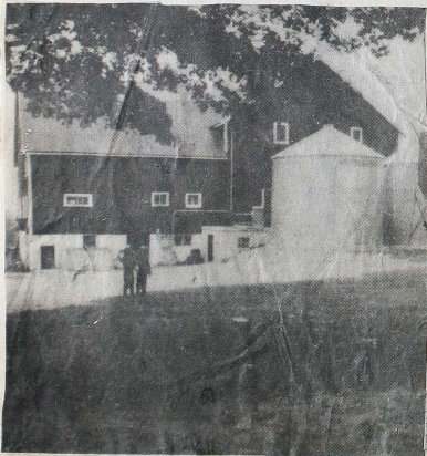
The barn of Dennis Robinson before it was completely gutted by fire last Tuesday, May 19.
