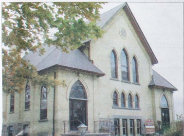
Above: Chalmers Community Congregational Church, outside of Armow. One of the contractors who built the church, George Conley, also designed and built the beach pavilion in Kincardine. The pavilion is also on display for Doors Open.
