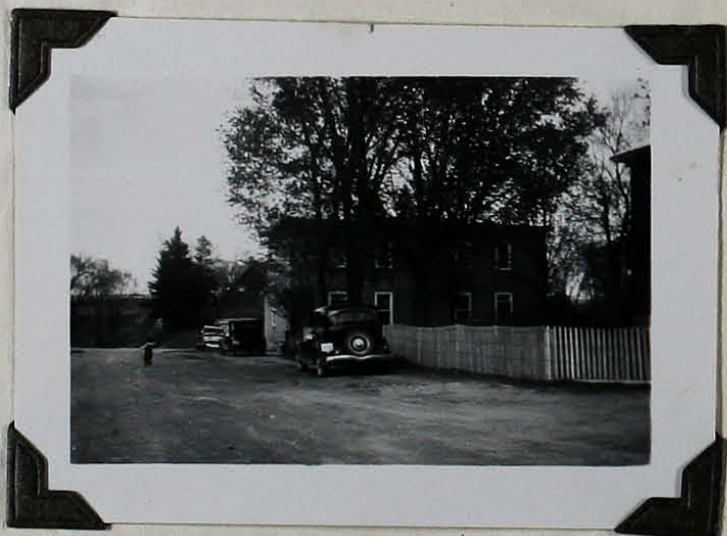
former B. V. Cheese factory now double dwelling house near Admaston Station. 1947
