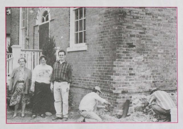
As their millennium project, the Vittoria Women's Institute initiated a \$30,000 restoration of their historic Town Hall where the Branch meets regularly. The restoration included repairs to the fieldstone foundation, repointing of the original brickwork, reconstruction of the chimneys and repairs and painting of the original windows. On the interior, a dropped ceiling was removed revealing a unique scalloped design and the original colours,
