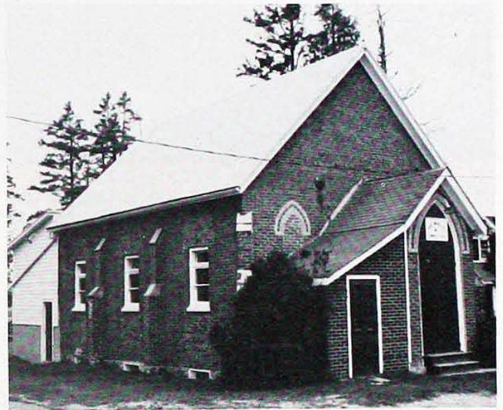
Former presbyterian church turned into a Community Hall owned and incorporated by The Maples WI, Dufferin South District.
