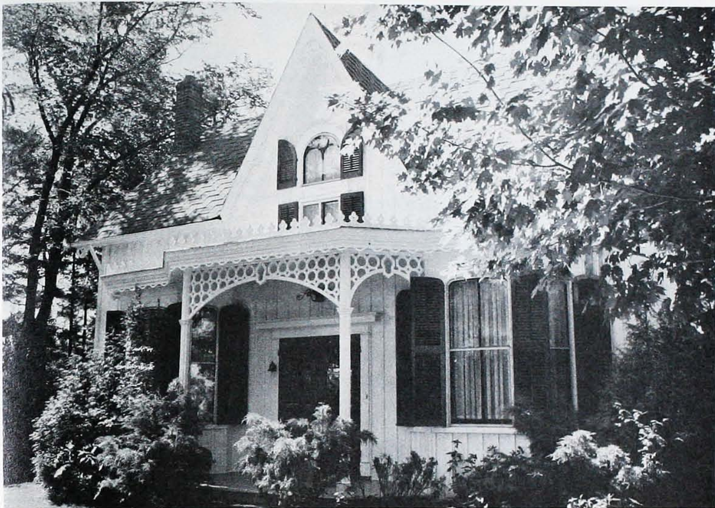
Pictured above is the new verandah on the Erland Lee Home, replica of the original. The front doors also were restored to their original style.
