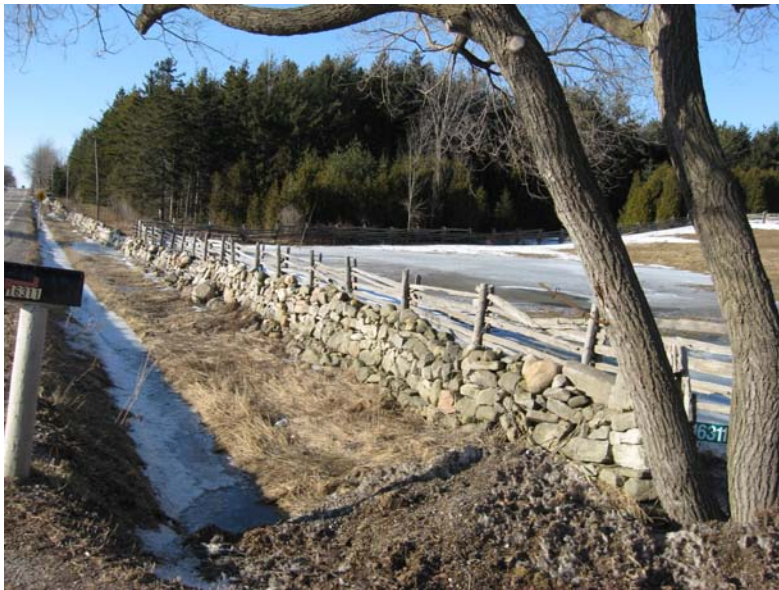
10 th Line, Esquesing – A dry stone wall backed up by a split rail fence. 2009 photo by J. M. Rowe
