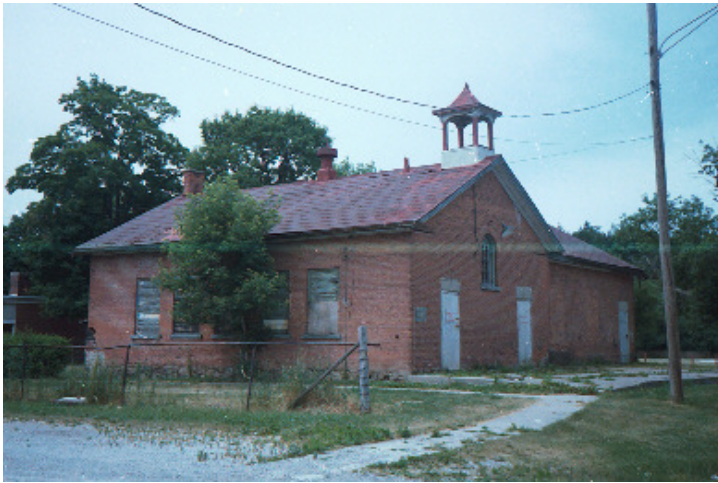
Norval Public School – SS#7 Esquesing built in 1859 with the 1874 addition. This picture was taken by John Somers in 1978, the year it was demolished. EHS12494
