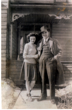
Photo confirms porch detail
