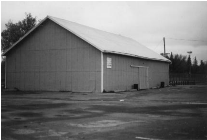
Acton Drill Shed (Fall Fair Poultry Barn) p946
