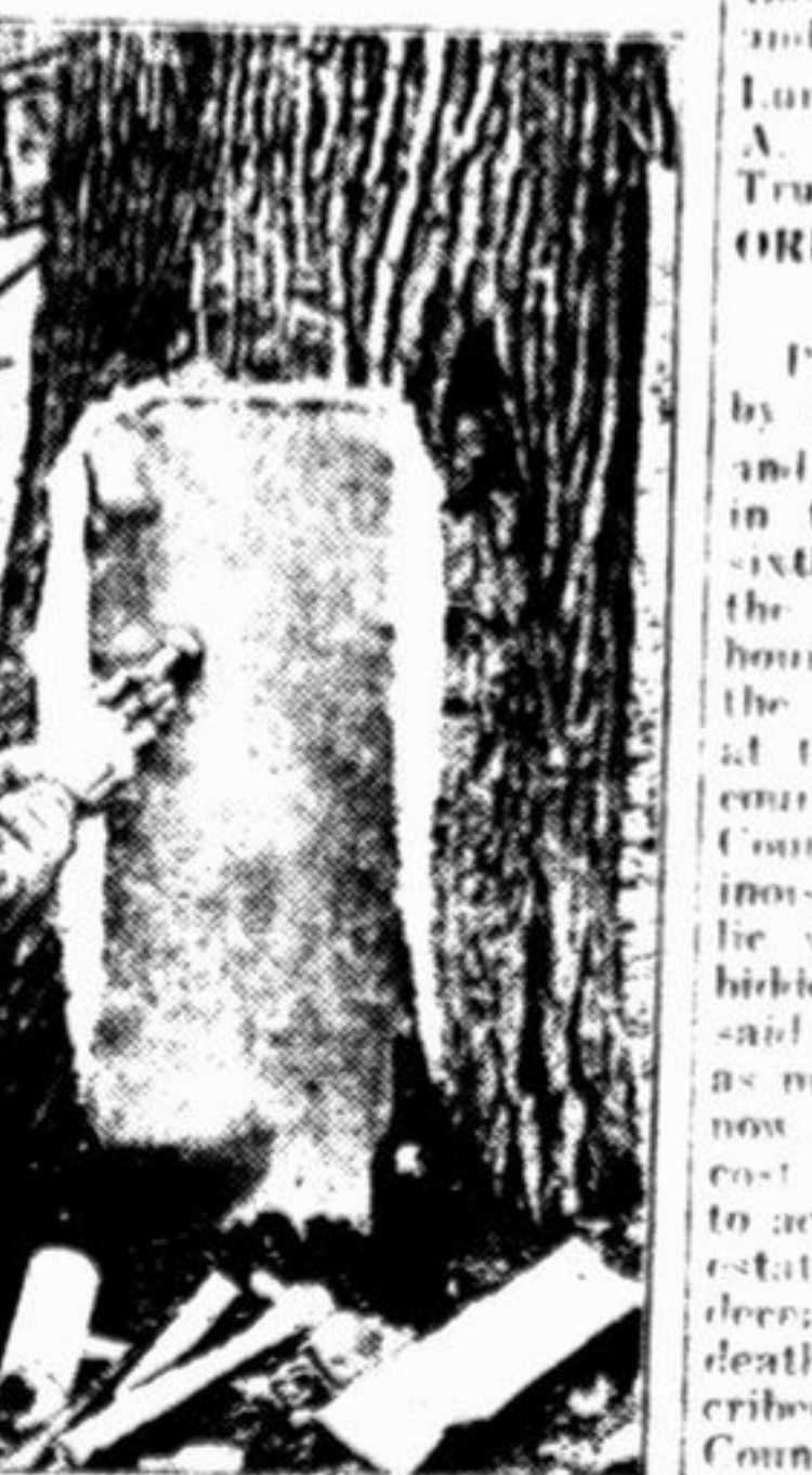
Decayed Stump of Gum Tree Prepared for Filling, Fumigated and Painted.
