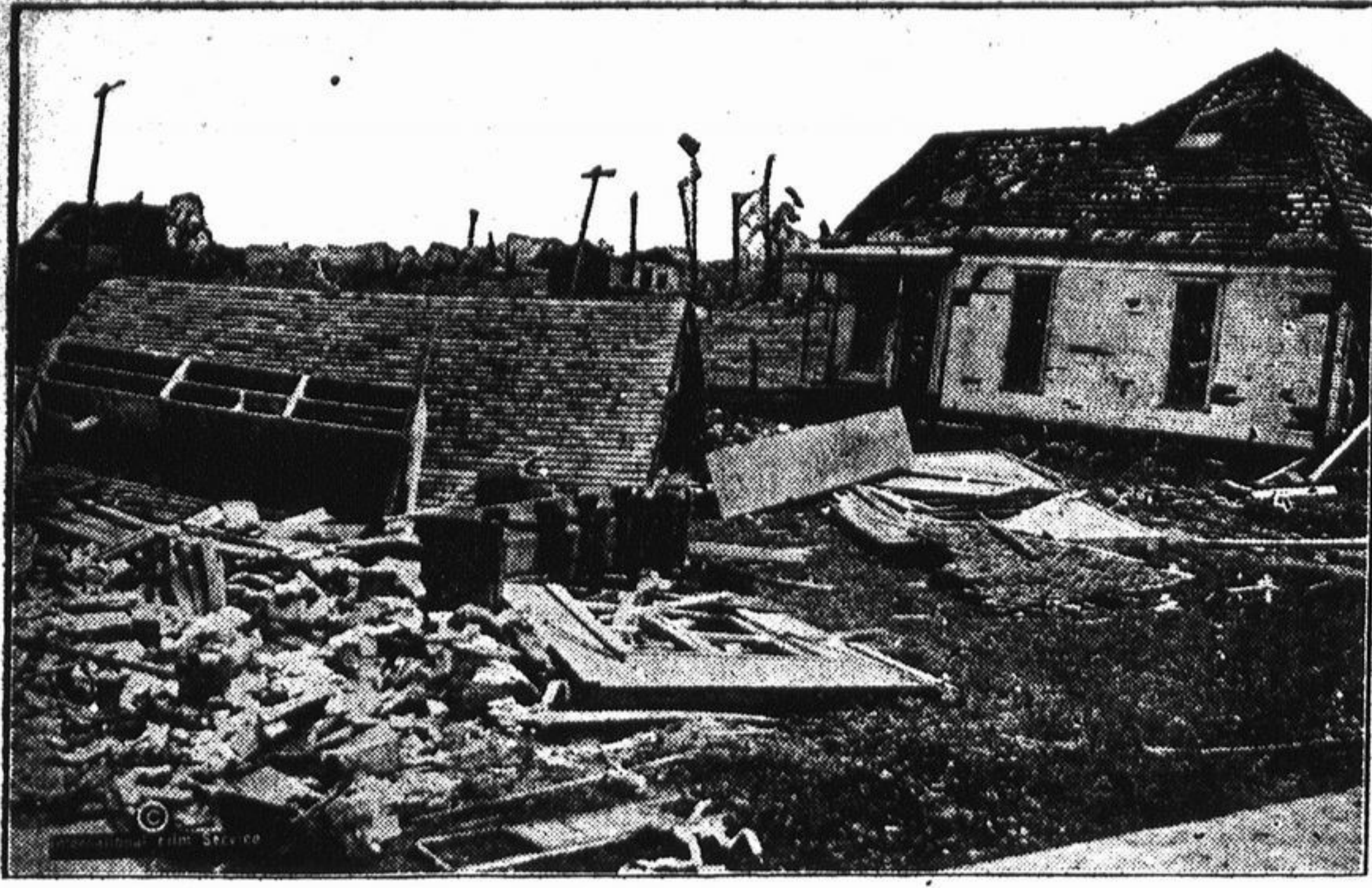
This scene on Thirteenth street, Mattoon, gives a vivid idea of the results of the terrific tornadoes that swept through central Illinois, killing about 180 persons and doing millions of dollars' worth of damage.
