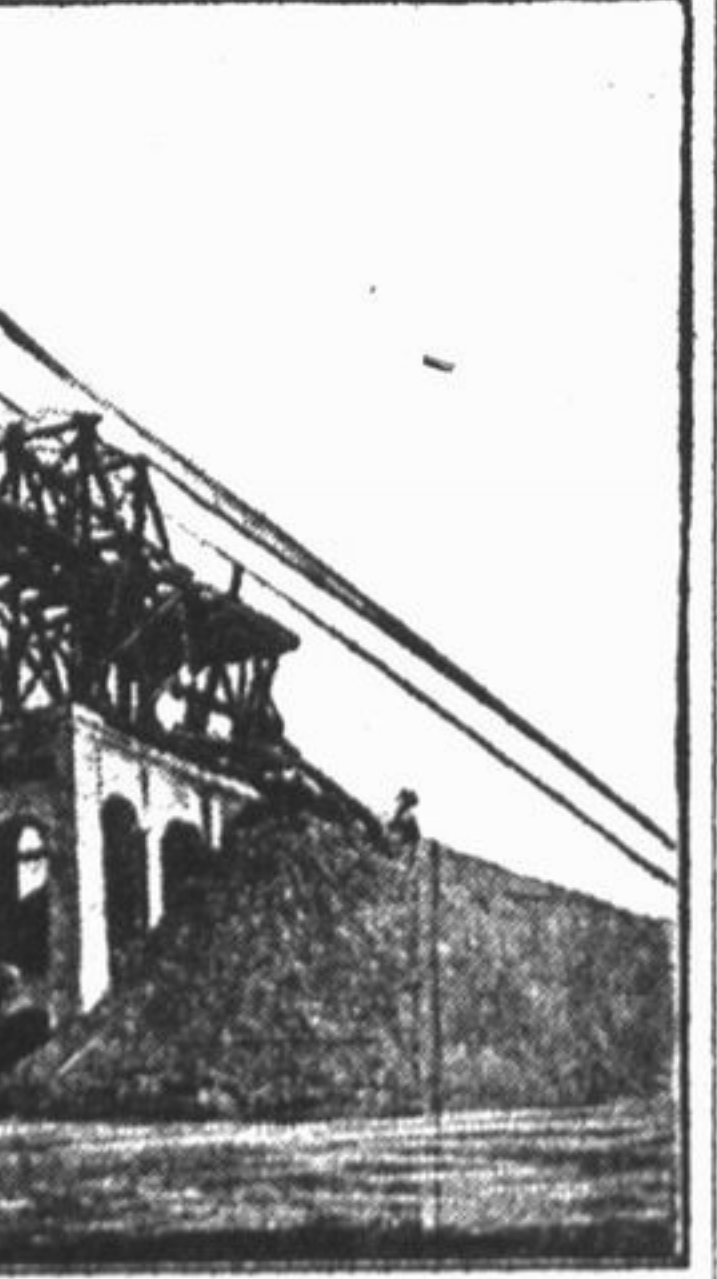
The Wooden Cantilever Traveler in Use Beginning the Erection of the Viaduct at Lewiston, Mont.
