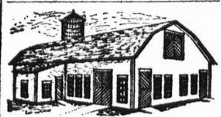
EXTERIOR VIEW OF BARN.
