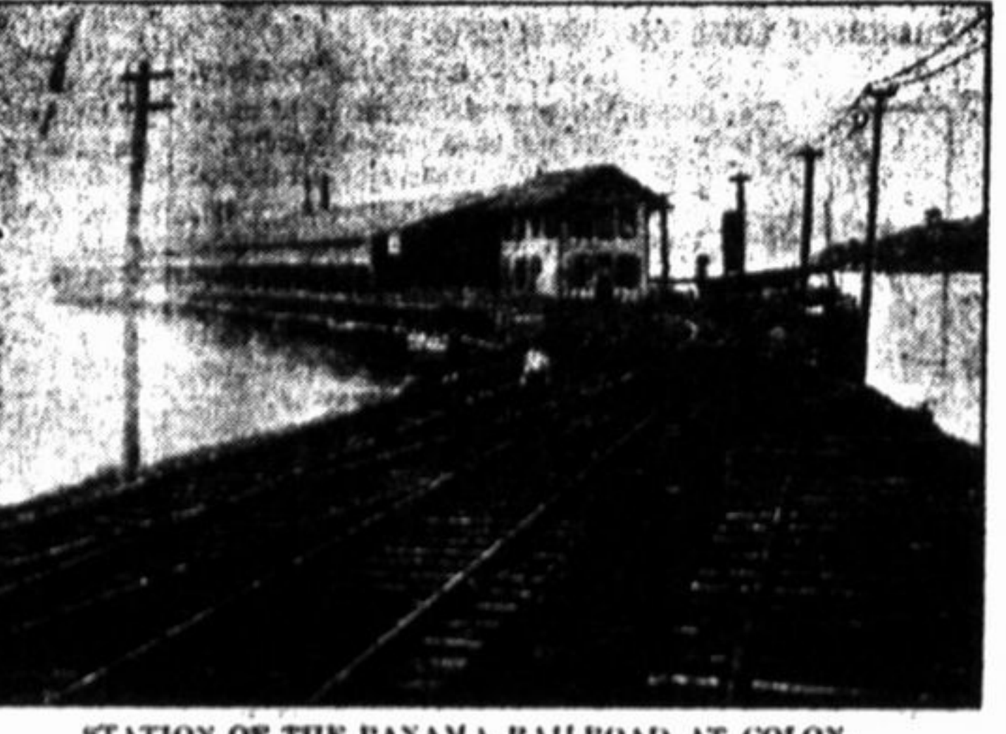
STATION OF THE PANAMA RAILROAD AT COLON.
