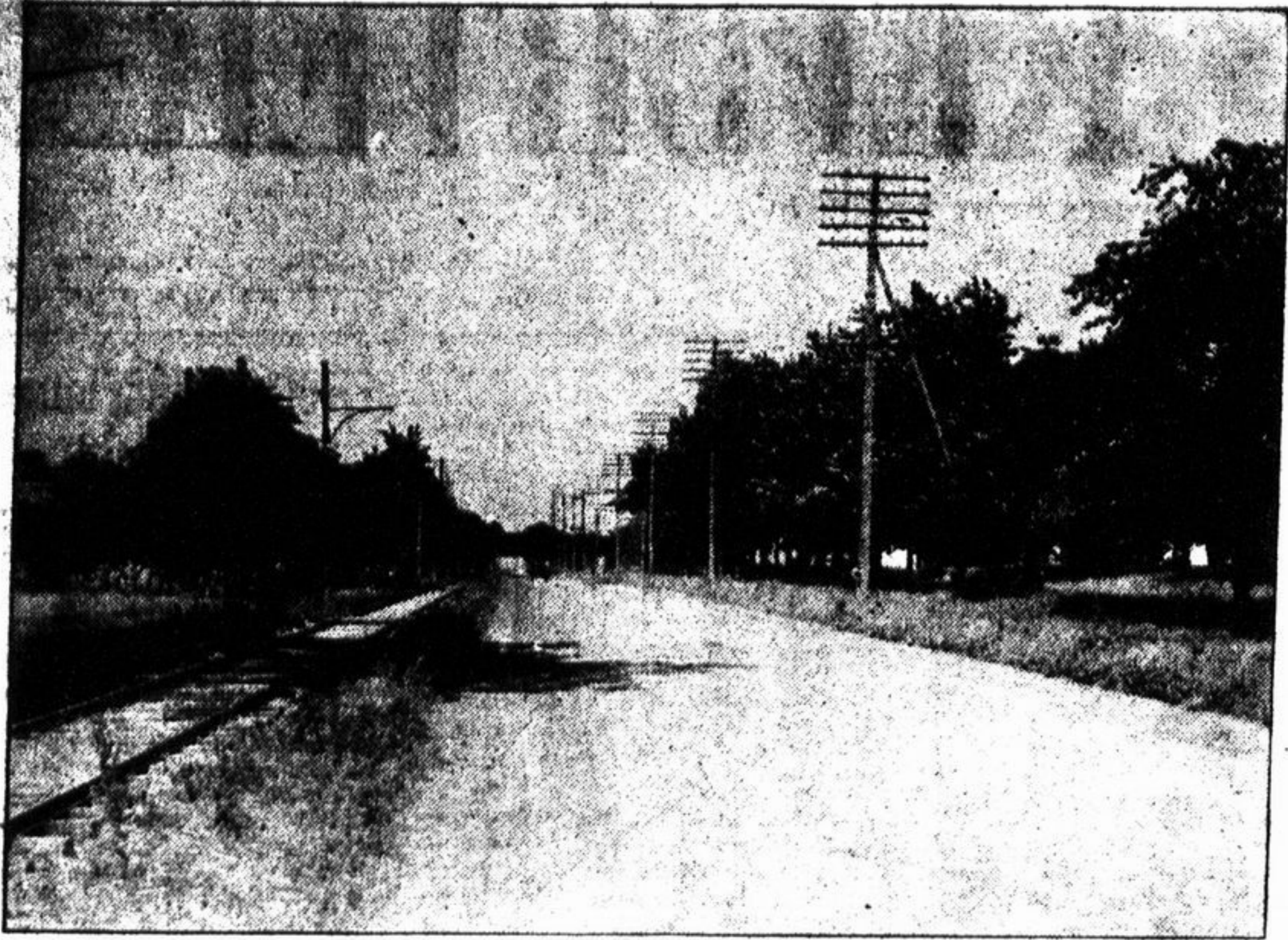
Williamsville Road, Erie County, New York, Just Out of Williamsville. This Road Was Treated with Tarvia in the Fall of 1907.
