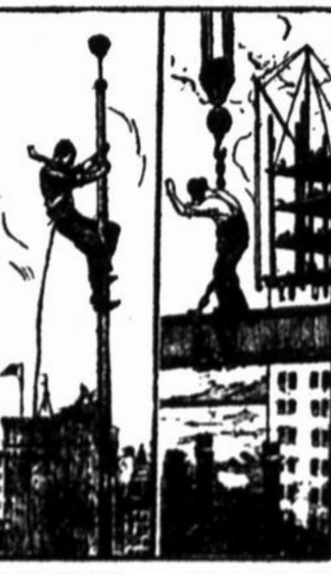
THE STEEPJACK. THE IRONWORKER.
