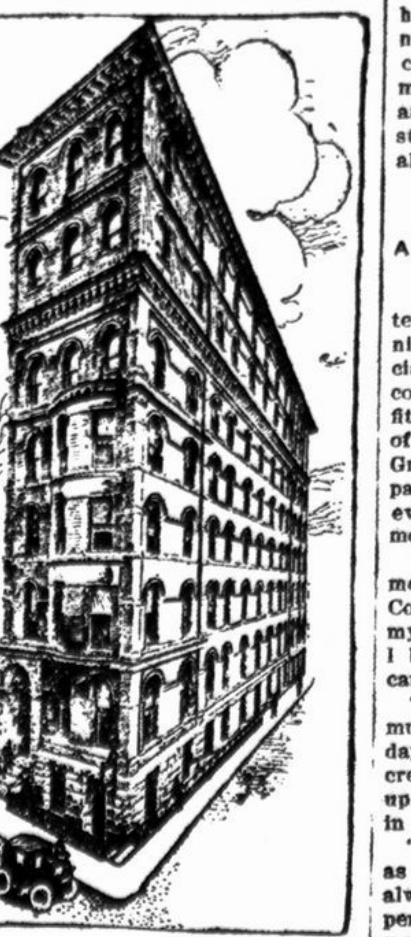
Where the fire started at 11 a. m. Sunday, Feb. 7.
