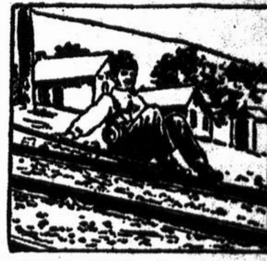
Method of Silding Down the Rail. notch is cut, which fits on the rail. On the shoe is rivetted a small square board—the miner's seat.
