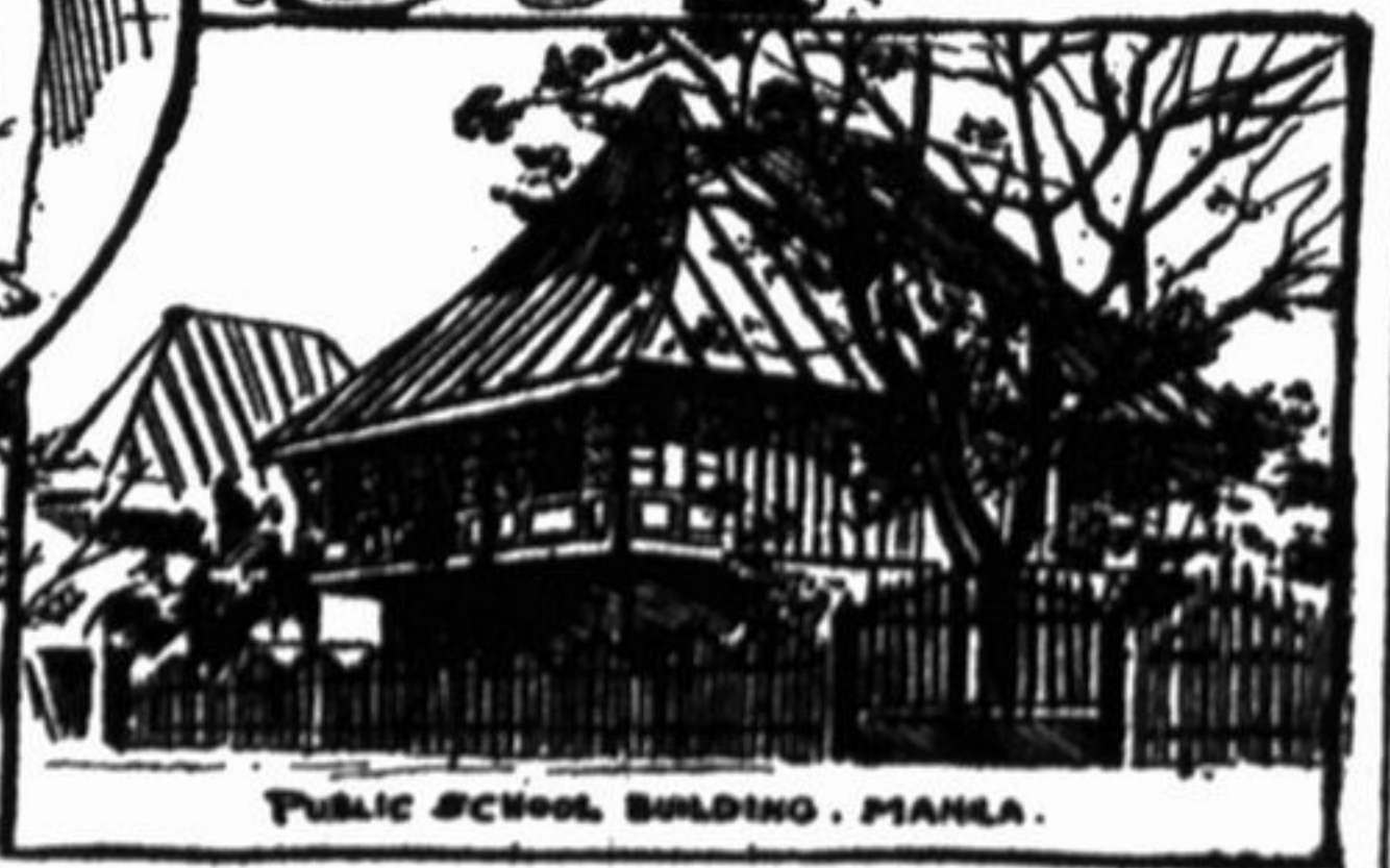
PUBLIC SCHOOL BUILDING - MANILA.
