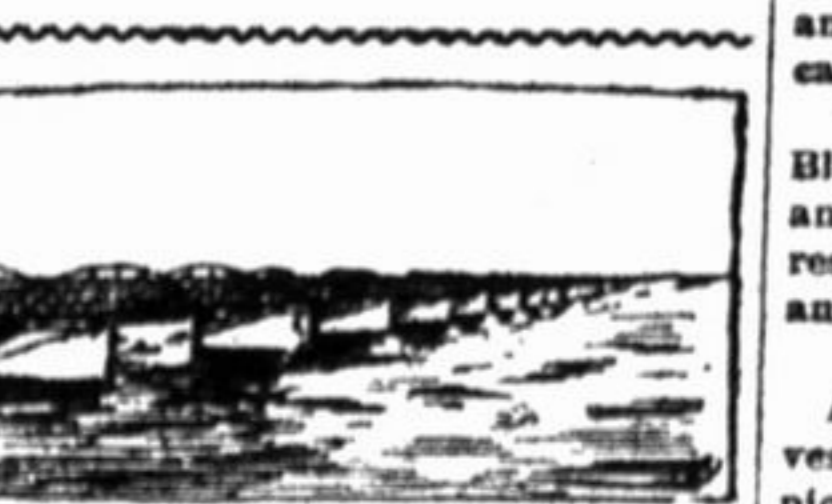
BRIDGE OVER GALVESTON BAY.
