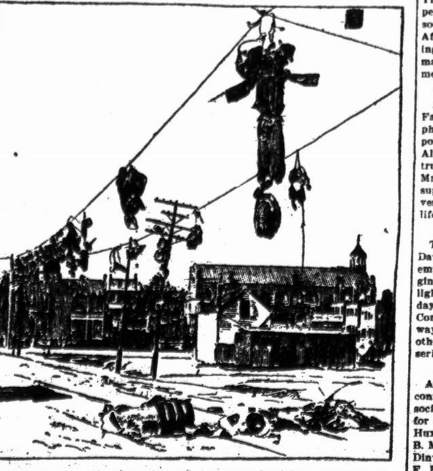
TROLLEY WIRE AND STREET OBSTRUCTIONS ON JEFFERSON AVENUE, NEAR UNIVERSITY STREET.
