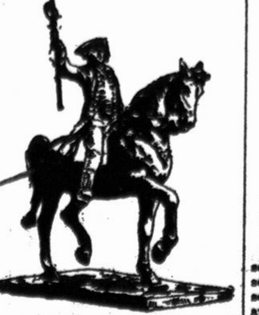
base is 26 feet 6 inches high, 24 feet wide and 18 feet 9 inches in depth.
