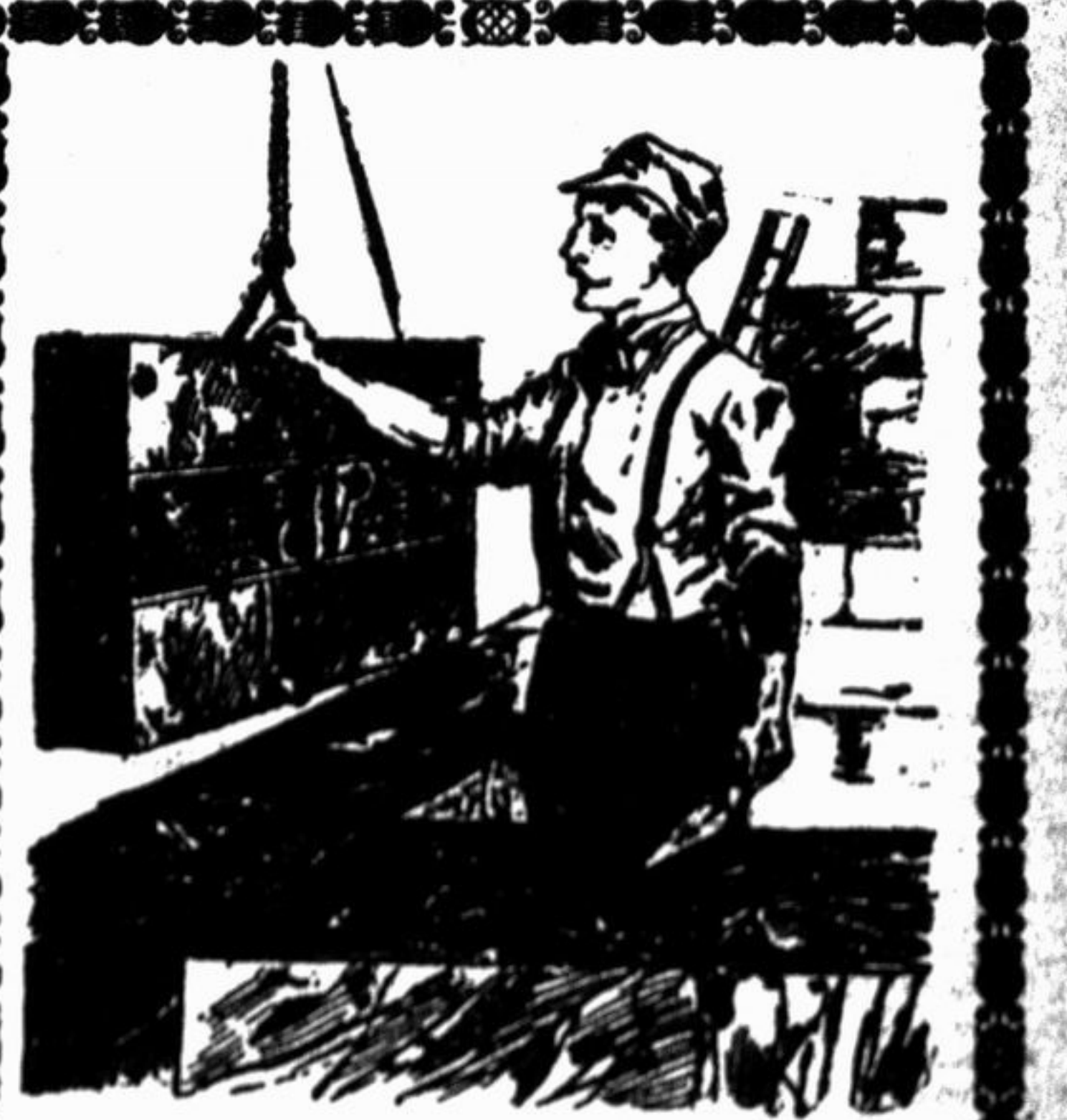
"A Good Foundation."
