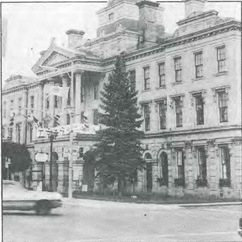
Two views of Cobourg's Victoria Hall: an 11-year overhaul.
