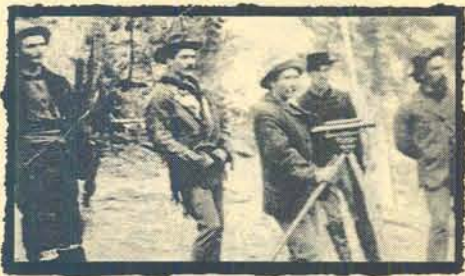
This Canadian Pacific Railway survey party is typical of those that Fleming would have visited as supervising engineer of the coast-to-coast CP survey.
